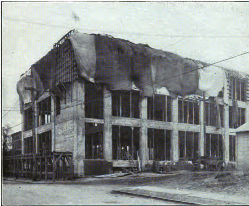
FIG. 8.—CANVAS HOUSING PROTECTING FRESH CONCRETE.
